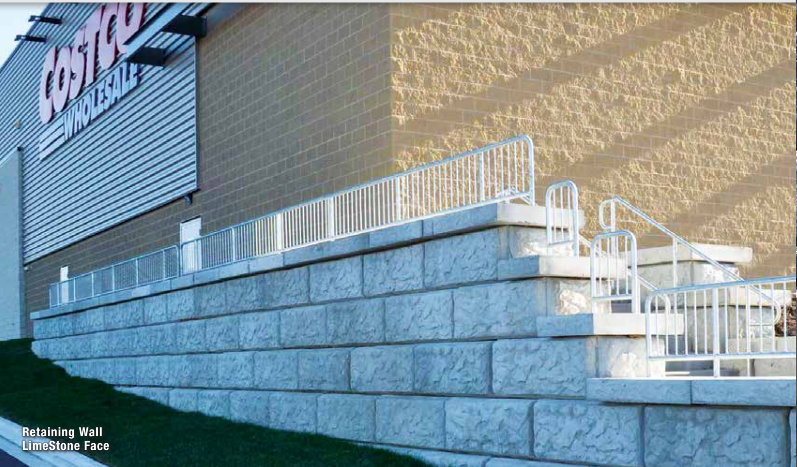
Retaining Wall CobbleStone Face / Stained
